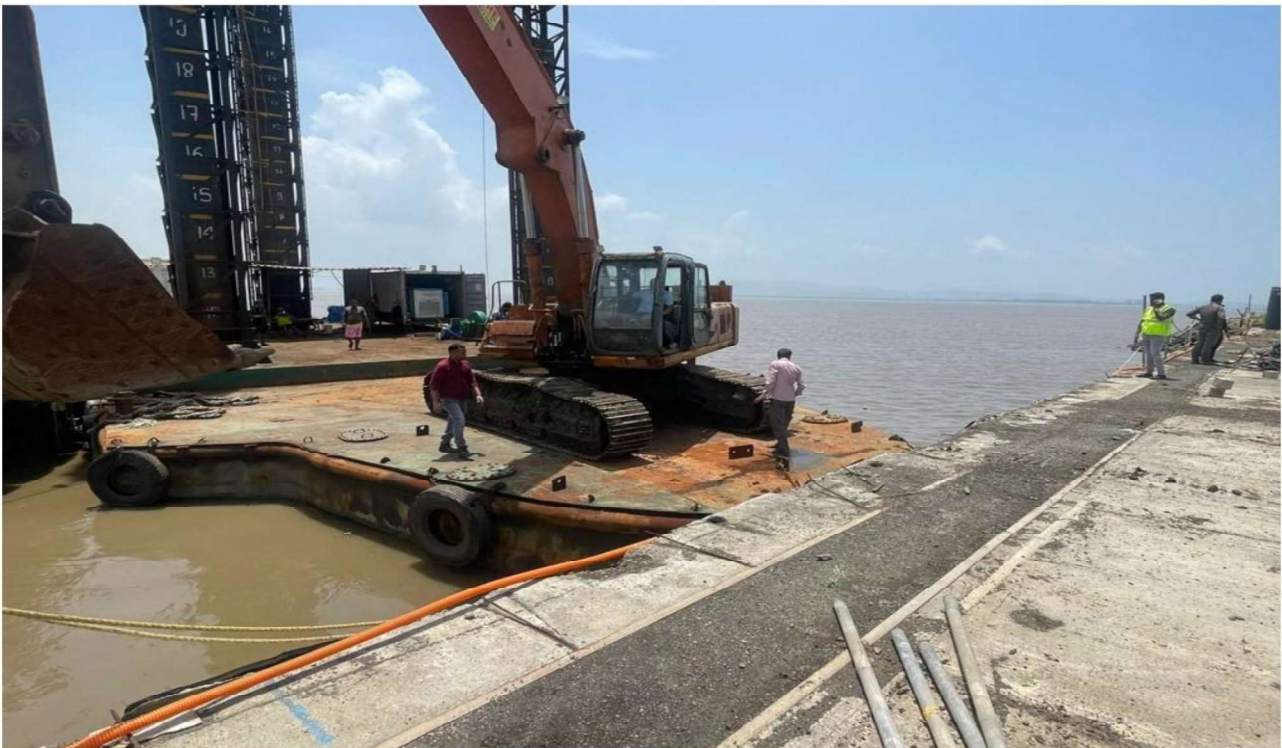
Maintenance Dredging Operations (above and below)
