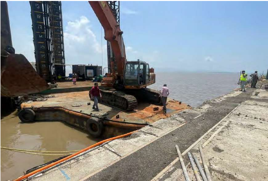
Maintenance Dredging Operations (above and below)
